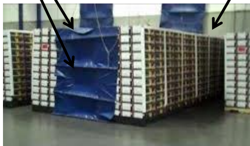
Picture of a forced air cooling tunnel
