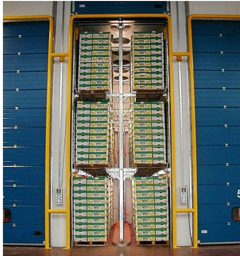
Fixed Forced Air Cooling Tunnel
