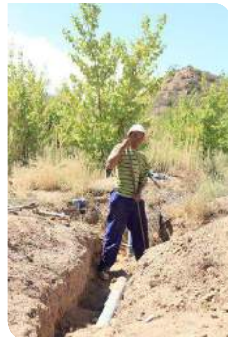
⬆ Nathan Volmink fixes a broken irrigation pipe.
